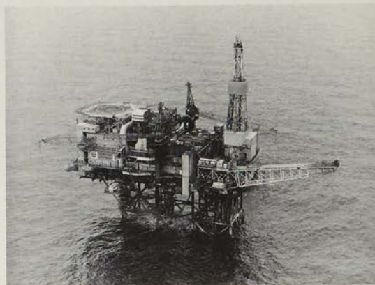
Chevron's Ninian Northern platform.
