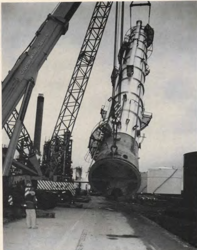
Deisohexaniser column being installed at Elf/Murco refinery in Milford Haven.
