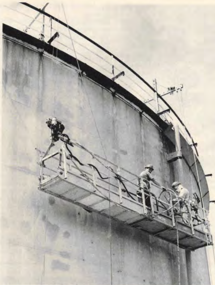
Vacuum spot blast cleaning tank shell from a 6 metre length cradle.
