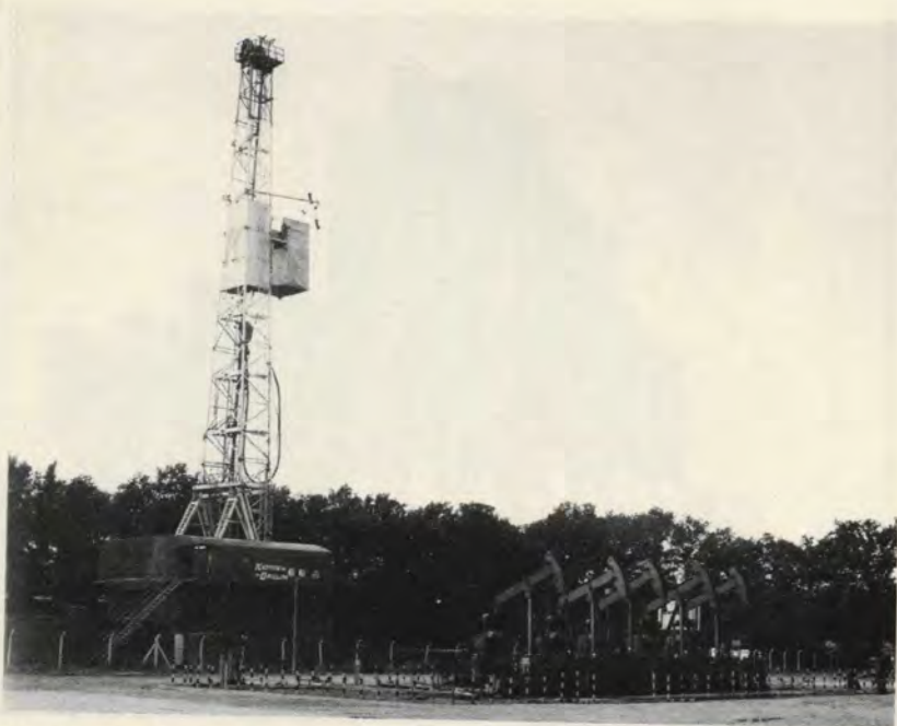
Development drilling at BP's Welton field
