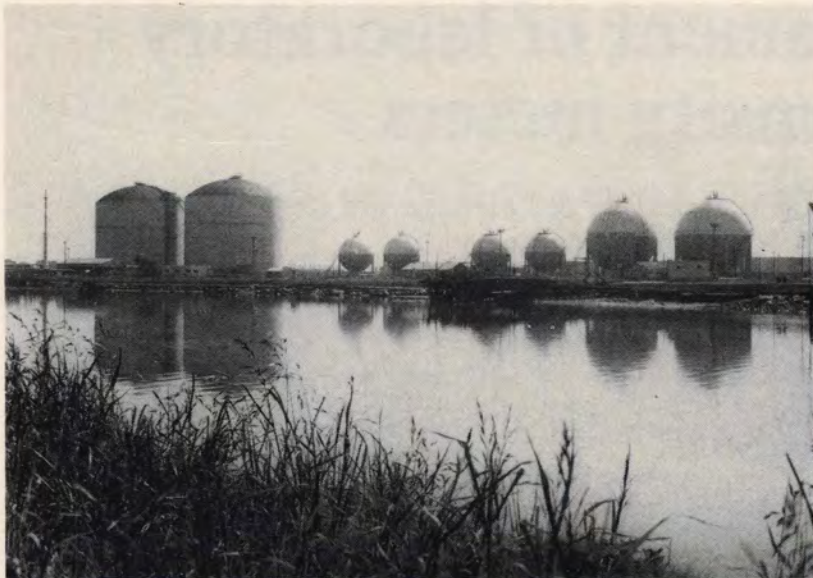
Dock Sud storage complex in Buenos Aires province.
