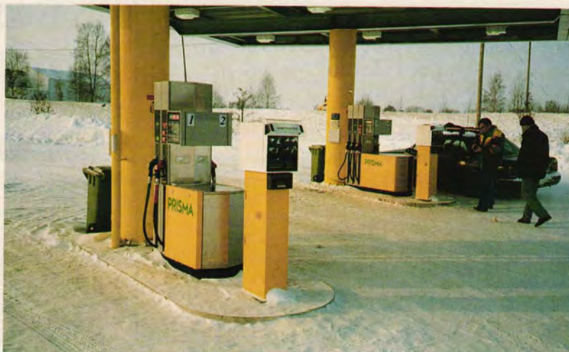
Photo 2: A fully automated service station in Sweden, developed by a supermarket chain as part of their standard layout. The station comprises AutoLane Multi Product Dispensers controlled by combined Bank Note Acceptors and Card Readers connected directly to a host computer.
