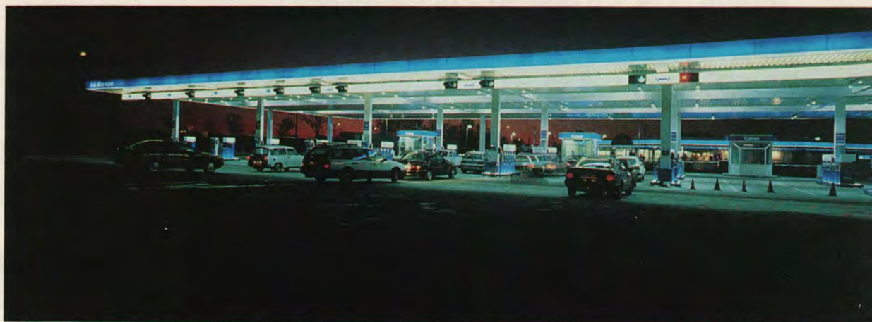
Photo 1: The Wilsdruff Service Station located in eastern Germany. One of the largest service stations in Europe. The 114 nozzles and eight point-of-sale tills are all interconnected by an optical fibre local area network. A comprehensive Back Office system (which is also connected to Aral's Head Office) helps the Manager to control the station and his 47 employees.
