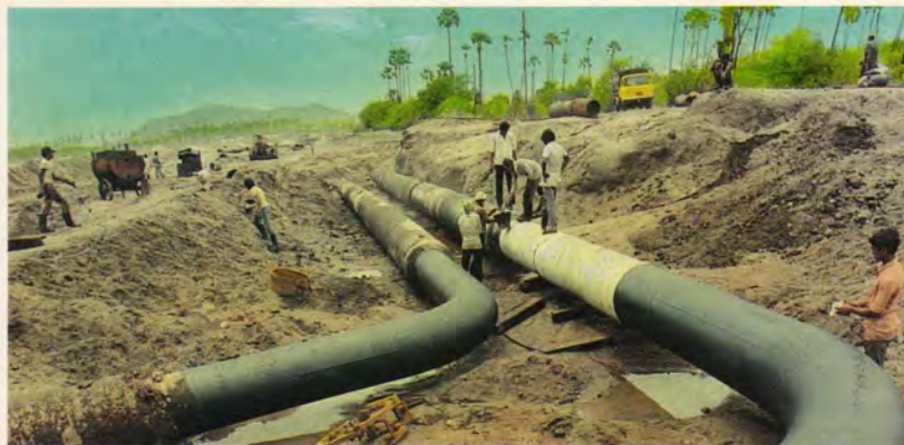
Piping work for Uran project
