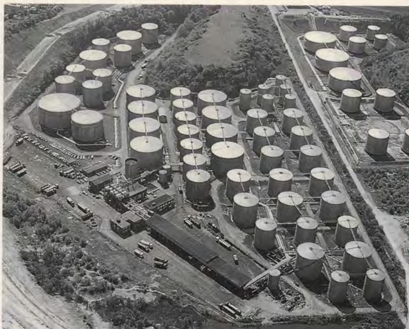
GATX's Eastham terminal
