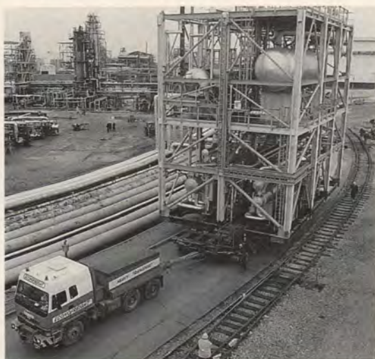
Transporting a prefabricated section within the refinery
