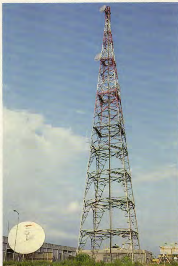
HBJ's microwave tower controlling gas trunkline operations.
