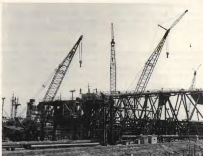
ONGC's first fixed platform under construction at Mazagon Dock
