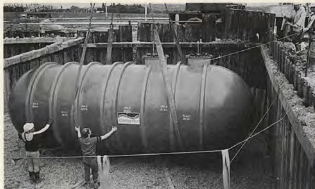
Installation of a glass-reinforced polyester storage tank on the M4
