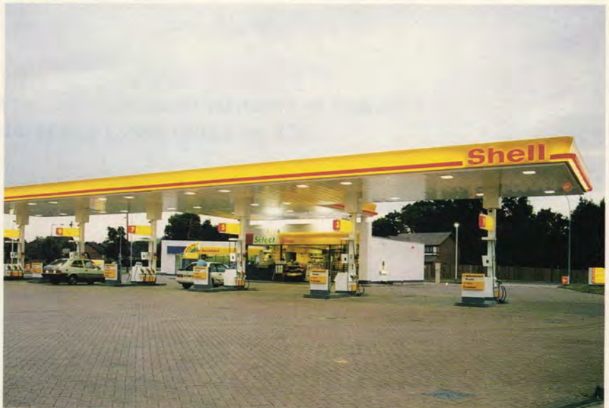
Horley service station after the redesign
