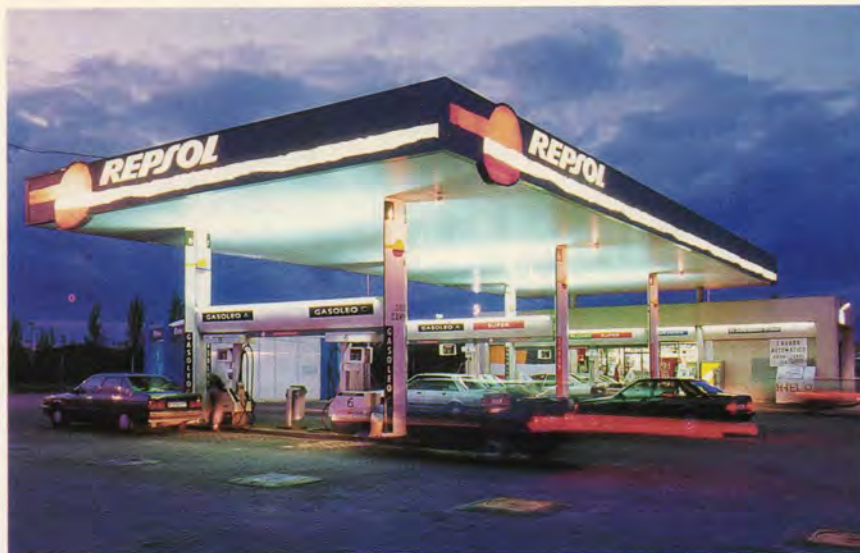
A Repsol service station
