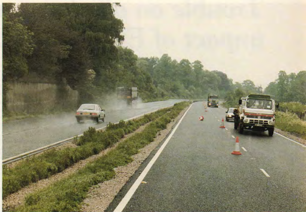
The A38 road near Burton on Trent on a wet day. Lefthand carriageway — hot-rolled asphalt; righthand carriageway — trials of new Shell bitumen.
