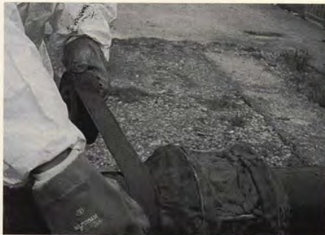
Premtape is cold-applied for anti-corrosion and water-proofing of pipes
