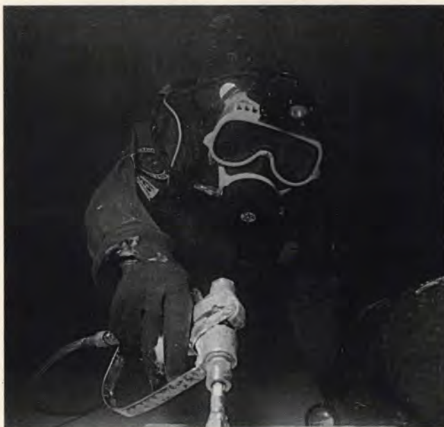
Alocit Aquacoat can be applied to wet and oily surfaces underwater
