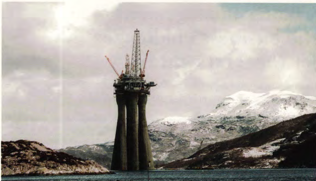
Last month the 472 metre-high concrete and steel platform was towed from Stavanger to the Troll field. (Photo courtesy of Norske Shell)
