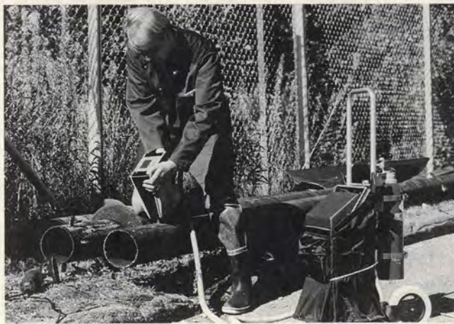
Portable optical emission analyser claimed to be the world's smallest
