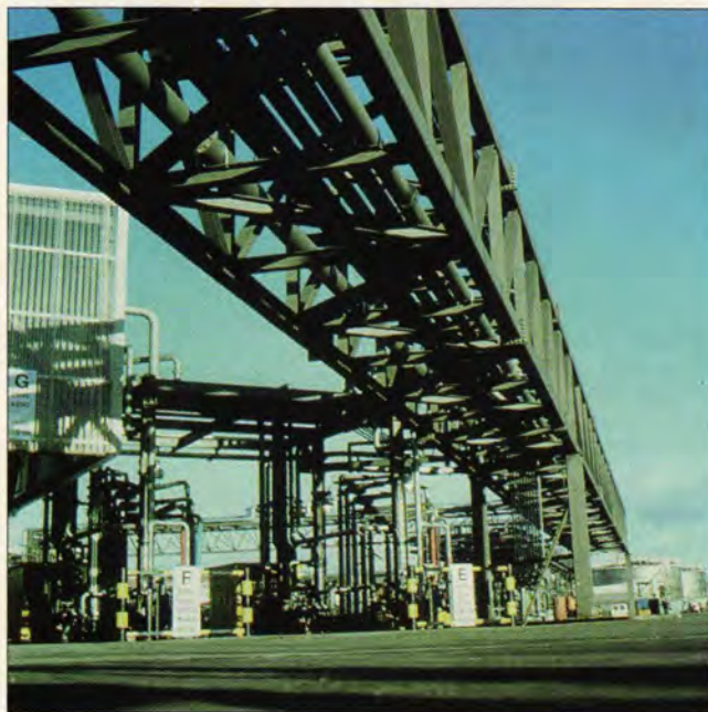
Kuwait Petroleum invests £5.7 million in new Scottish terminal
