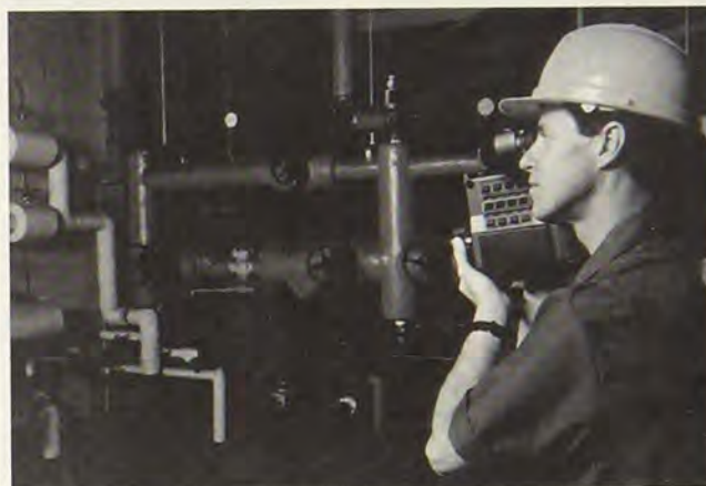
Inspecting for 'hot spots' at sea with a Thermovision 450
