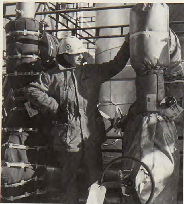
In the event of fire, the rubber jacket transforms into a hard shell
