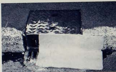
Mats can be bent to seal vertical drain inlets
