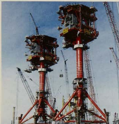
The Davy and Bessemer gas fields use Amoco's lightweight and cost-saving AMOSS platform design
