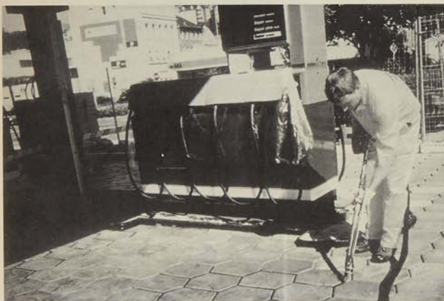
Application of a polysulfide sealant at a service station
