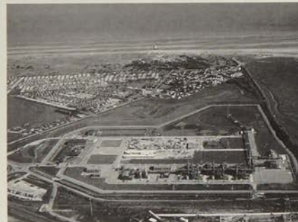
Point of Ayr gas processing terminal
