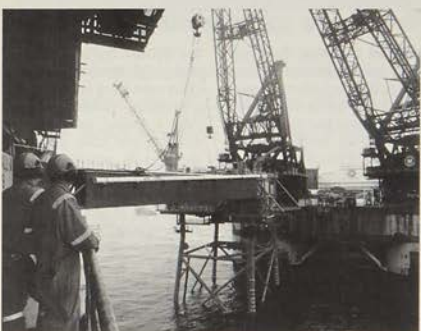
Valhall's new wellhead manoeuvres into position
