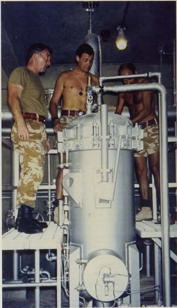
Operation Yarra: Overhaul of filtration system on permanent fuel installation in Bahrain
