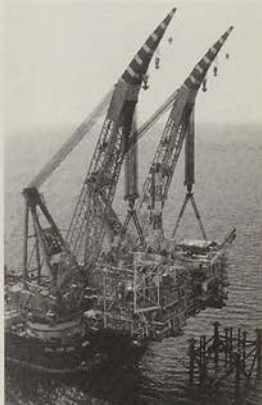
Installing Andrew's integrated deck
