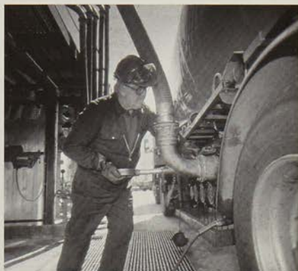
New bottom loading facility at Immingham
