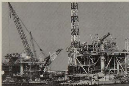
Trent and Tyne decks under construction at Lowestoft
