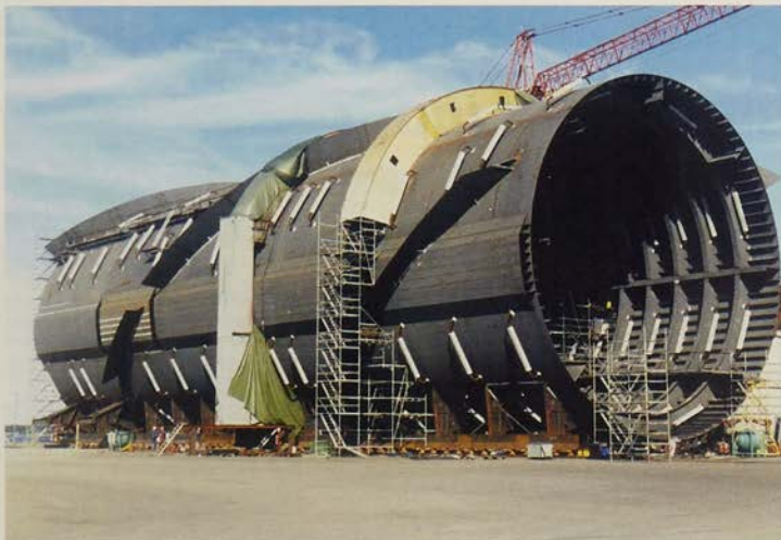
The world's first Spar production platform under construction by Aker Rauma Offshore
