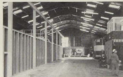
Cuttings processing facility
