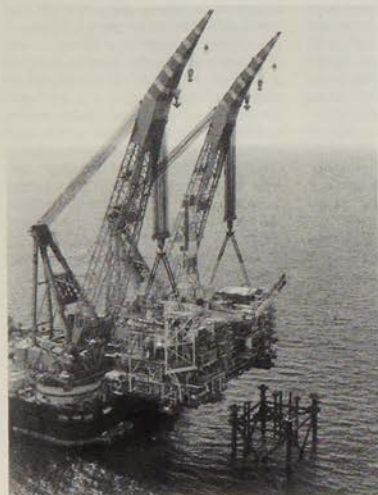
Installing Andrew's integrated deck
