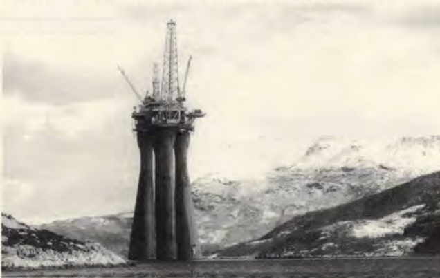
Troll platform tow-out (photo courtesy of Norske Shell)
