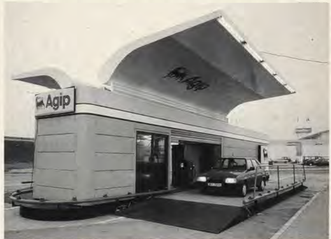
The 'wing' canopies on the new mobile station fold down for added security when the facility is not in use
