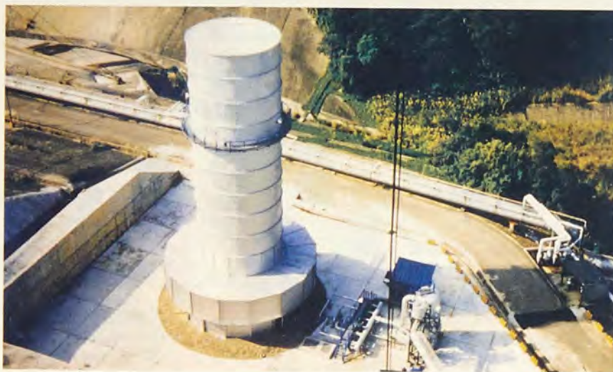
Designed to destroy 100 tonnes per hour of volatile organic compounds, this smokeless steam-free enclosed flare is located in a refinery near a major international airport, surrounded by dense urban development
