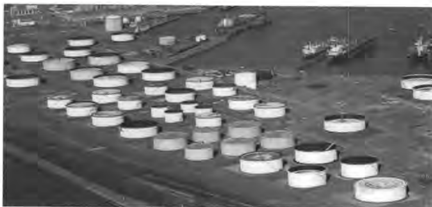
Storage installation with both fixed- and floating- roof tankage
