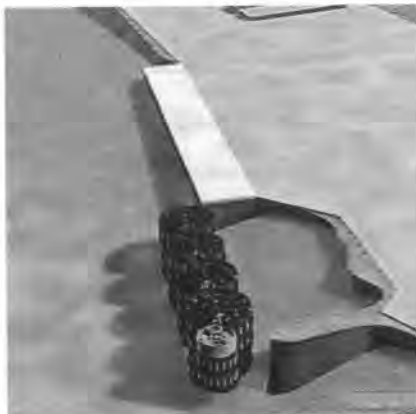
Spar 'slices' positioned for quay extension
