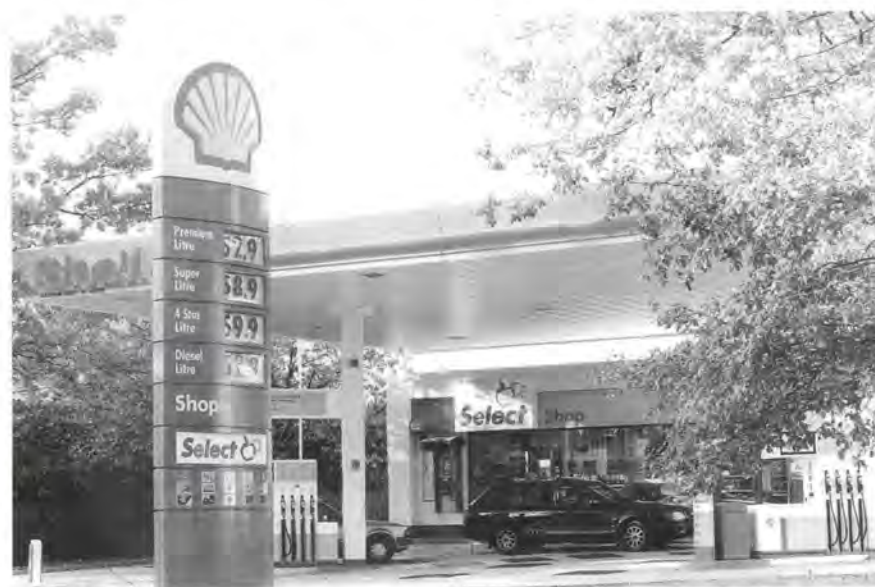
One of the 200 Shell service stations built and refurbished under its three-year agreement with David McLean Contractors
