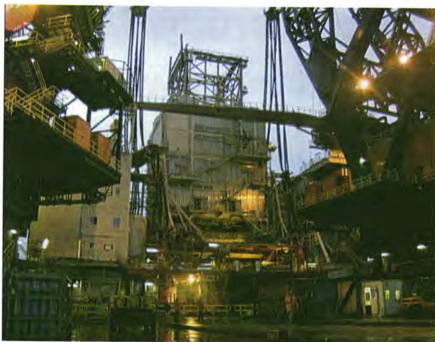
Jotun B wellhead platform topsides (8,500 tonnes) being installed by Heerema Marine Contractors' Thialf floating crane
