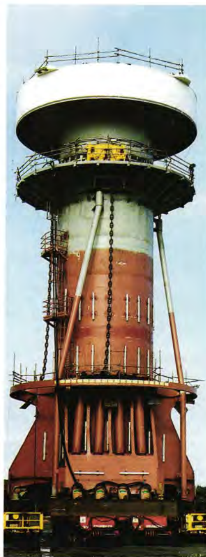
Load out of Jotun mooring current and anchor spider from Lewis Offshore's Stornoway facility
