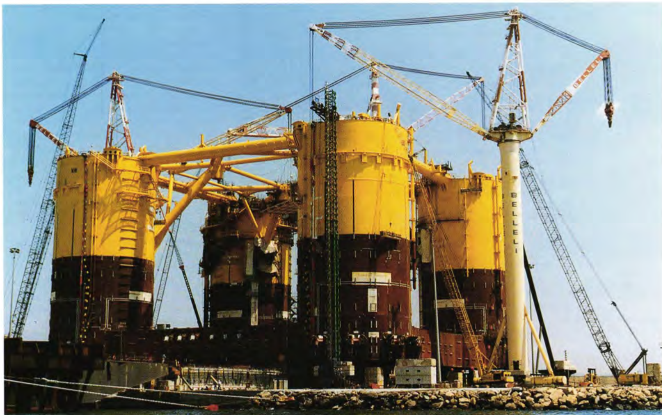
Ursa TLP hull, delivered to Shell by Belleli in June 1998
