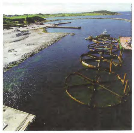
Shell's Brent Spar has now been dismantled in Norway and sections of the hull used as the foundation for a deep-water quay near Stavanger
