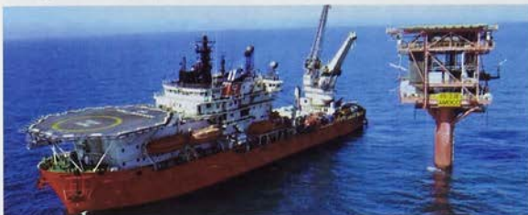
CSO Wellservicer alongside the Bessemer platform
