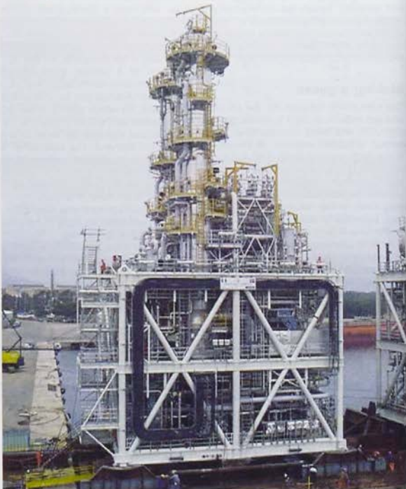
Intermare Sarda recently completed fabrication of the M20 stabilisation module for Statoil's Asgard B project
