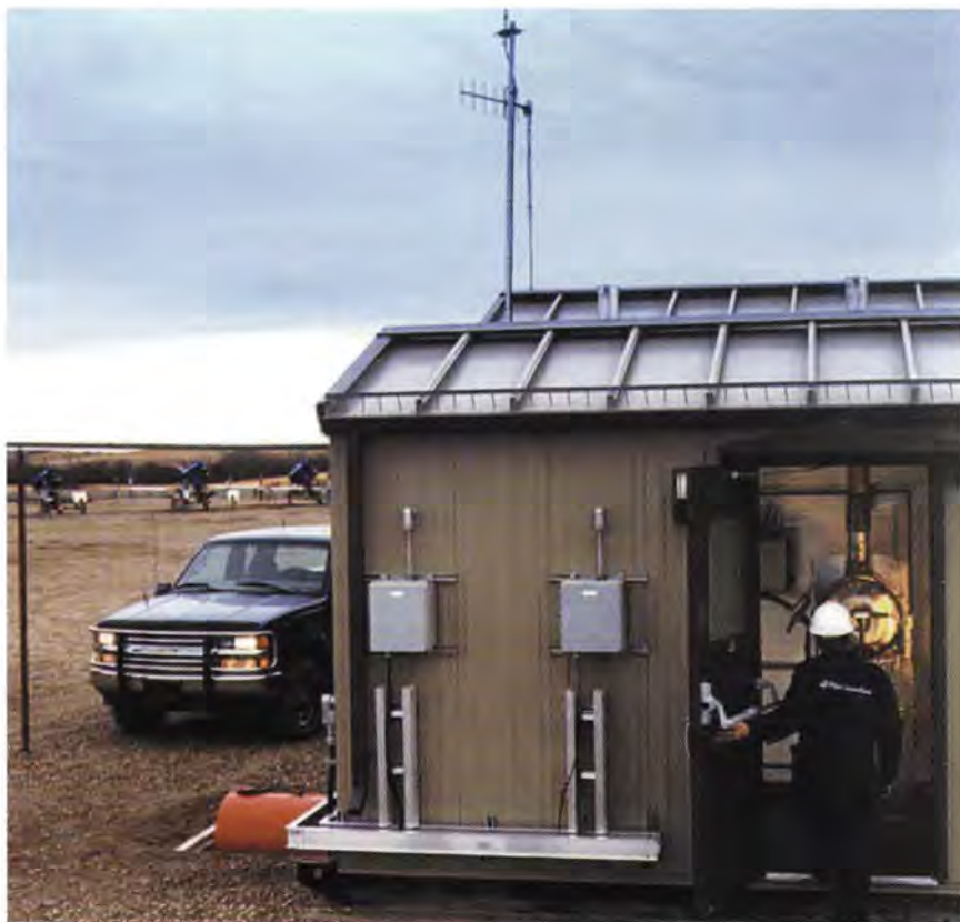
A PanCanadian operator stops to check two Capstone MicroTurbines™ installed in October 2000 at the company's Wainwright oil field. The turbines burn about 9,000 cf/d of natural gas, generating about 28 kW of electricity, sufficient to power the rotary oil well pumps seen in the background.
