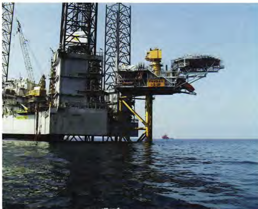
BP's Tambar platform is 'emissions-free.' Power, for example, is imported by subsea cable from Ula. Here, the jack-up Transocean Nordic prepares to start development drilling.
