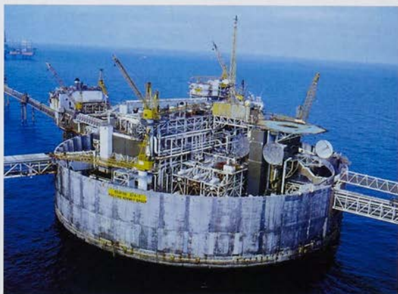
Phillips is tendering for removal of the Ekofisk Tank topsides. When this is completed, the tank's concrete base and protective wall will be left in place. Photo: PPC/NKjetil Alsvik
