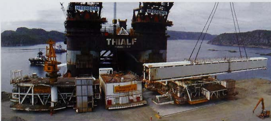
Crane-barge Thialf deposits the topside structures from Statoil's 2/4-S platform on the quay at Lyngdal Recycling's site in southern Norway. Photo: Sverre Dunseth/Statoil
