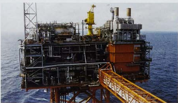
Captain's wellhead protector platform is bridge-linked to a process/utility platform.
