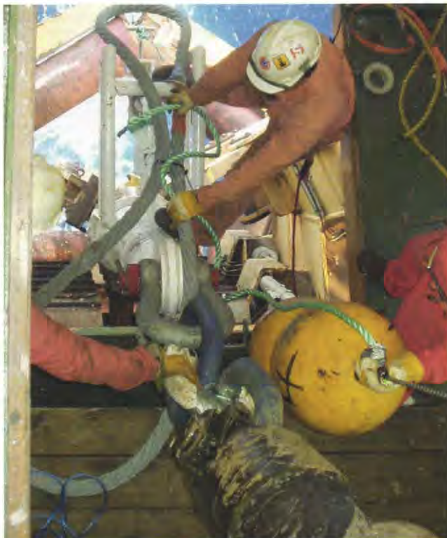
One of the in-field flowlines for the BG-operated West Delta Deep subsea development is readied for abandonment. A slack wire loop is attached to the abandonment and recovery head to facilitate flowline recovery for attachment to the pipeline end terminal
