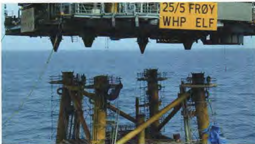
The Frøy topsides was removed by Heerema crane-barge Thialf in July 2002. TotalFinaElf still has hopes of finding a buyer for it
