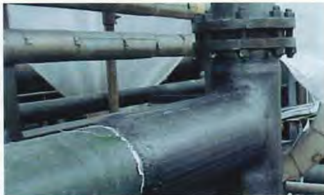
Composite wrap repair to tee pipe
