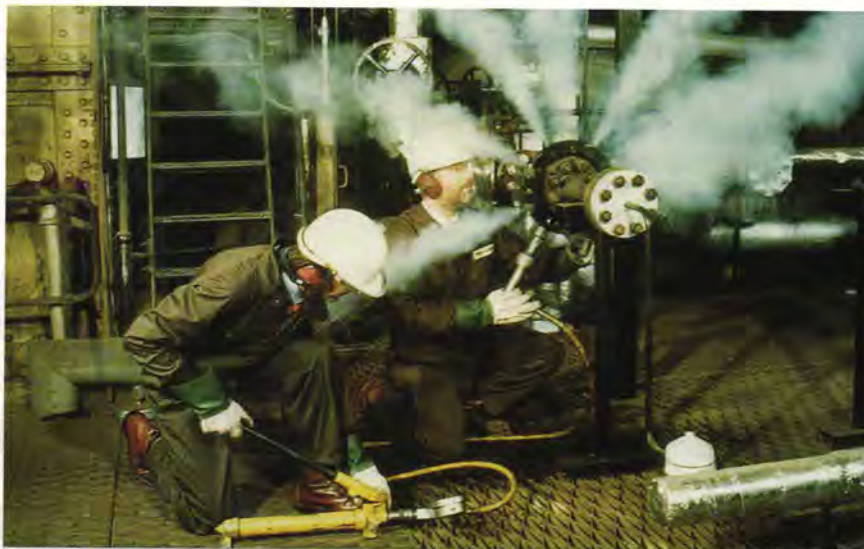
Furmanite leak sealing
