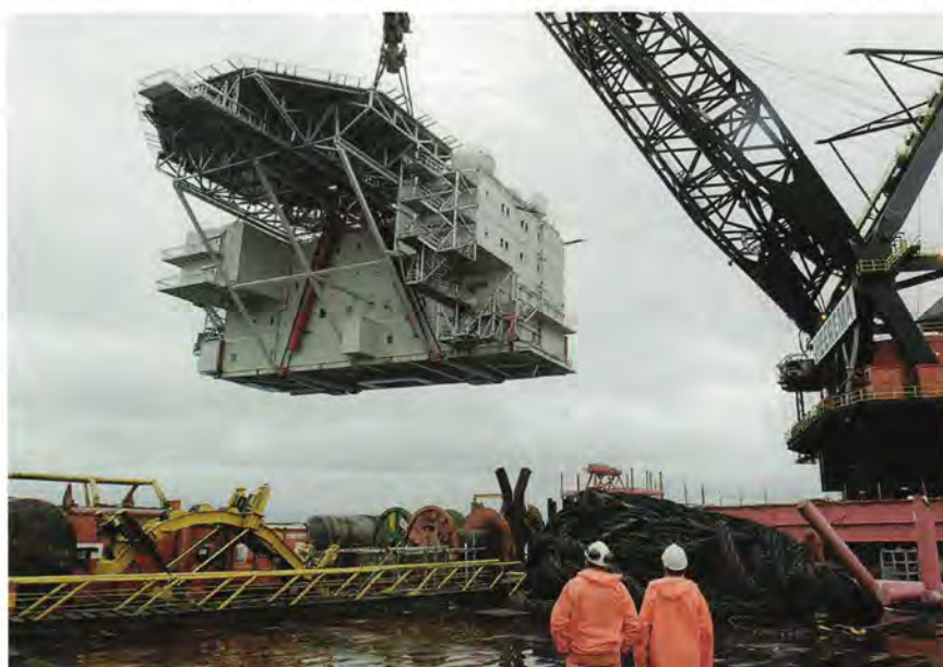
Offshore installation of the 120-man living quarters for Esso Norge's Ringhorne development in the North Sea, fabricated by Emtunga, delivered to Heerema Tonsberg in 2001.
