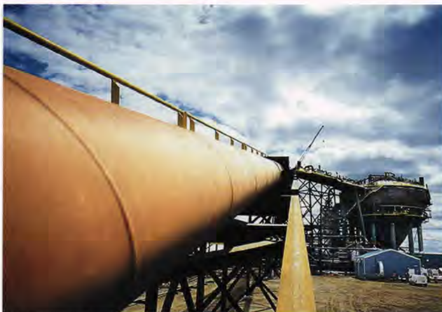
Hydrotransport pipeline leads to the aurora primary separation vessel
