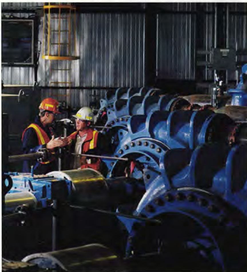
Froth booster pumps at the Aurora project
