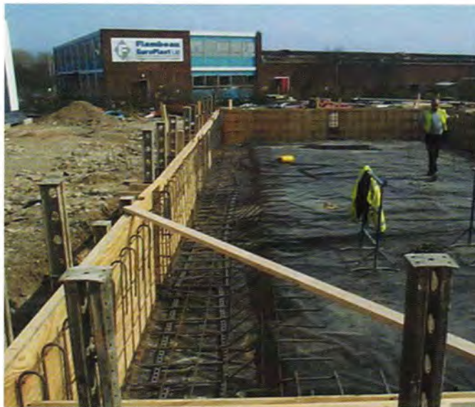
Top: The finished Tesco service station with the tank storage facility in the background. Above left: the foundations for the above ground storage tank being laid. Right: installation of the tanks
