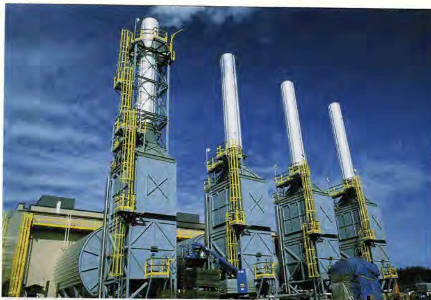
Petro-Canada's Mackay River site – four steam generators, a key component of producing bitumen using horizontal well pairs
