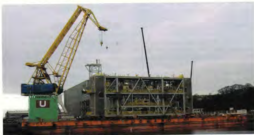
BP's Clair skid at Burntisland Fabrications yard
