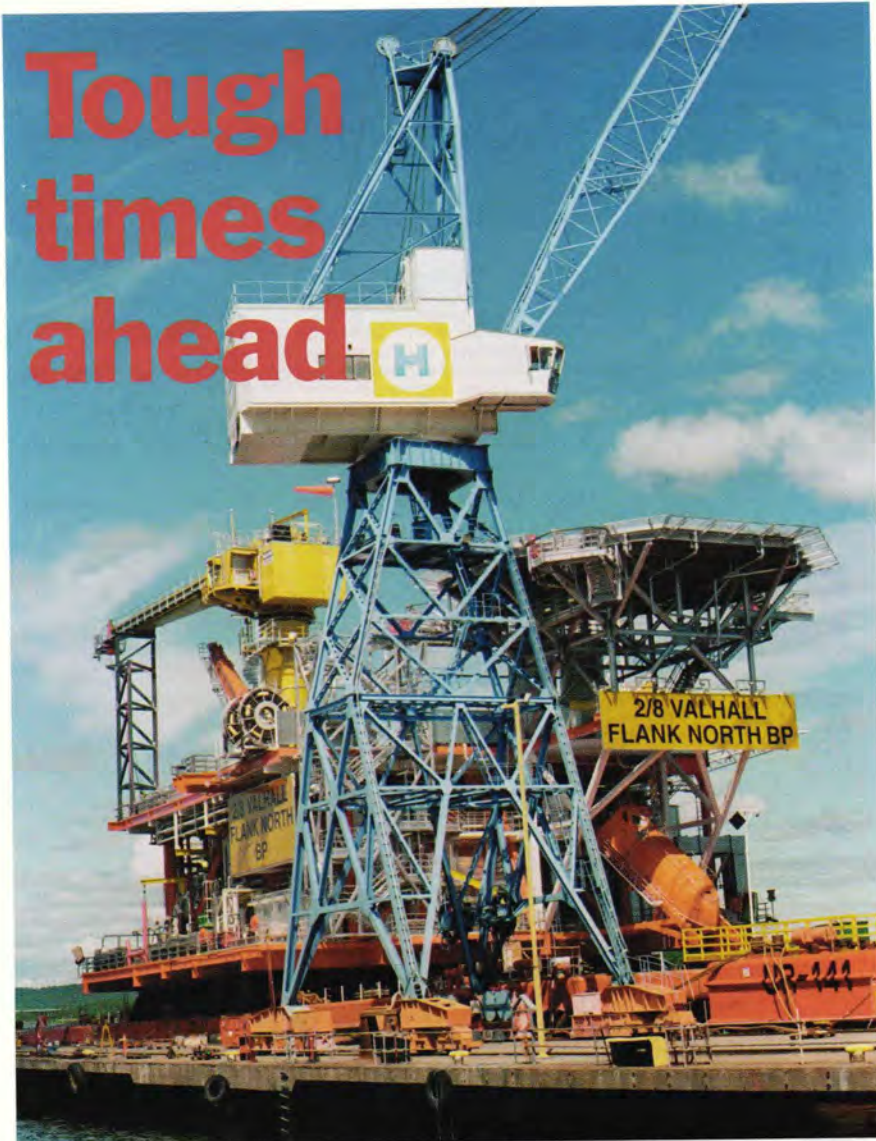
BP Valhall Flank development – North platform. EPCI contract for Heerema Tonsberg, delivered and installed July 2003
