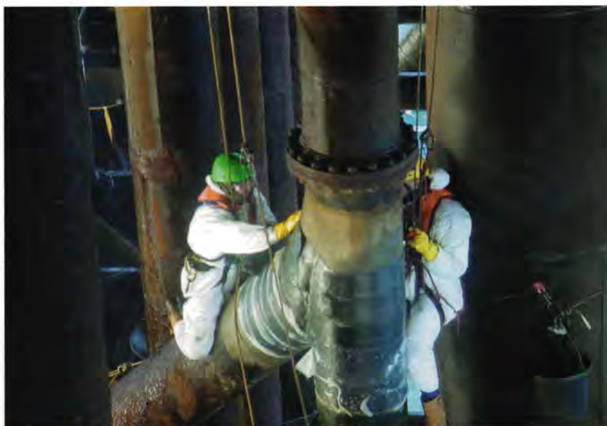
A repair to a riser on a North Sea production platform
