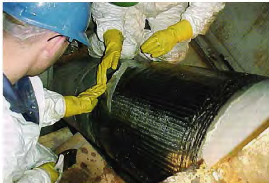
Application of resin composite to achieve a pipe repair
