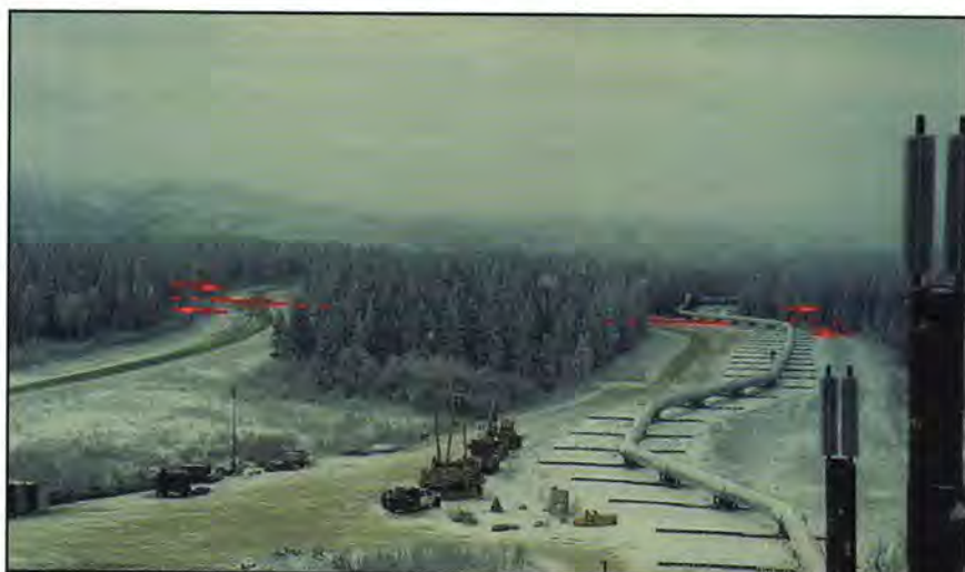
Figure 3: Denali fault, Alaska. Fault rupture by Richardson Highway beneath Alyeska pipeline. Red lines indicate location-direction of movement across fault. Pipeline N fault shifted W centre on horizontal sleeper rails
