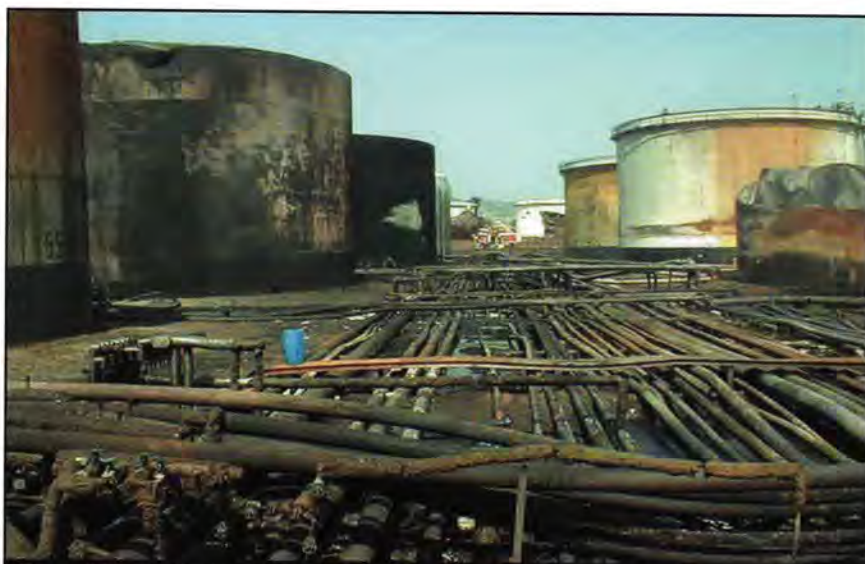
Figure 2: Burnt storage tanks and pipes at the Tupras refinery following the August 1999 Izmit (Kocaeli) earthquake in Turkey
