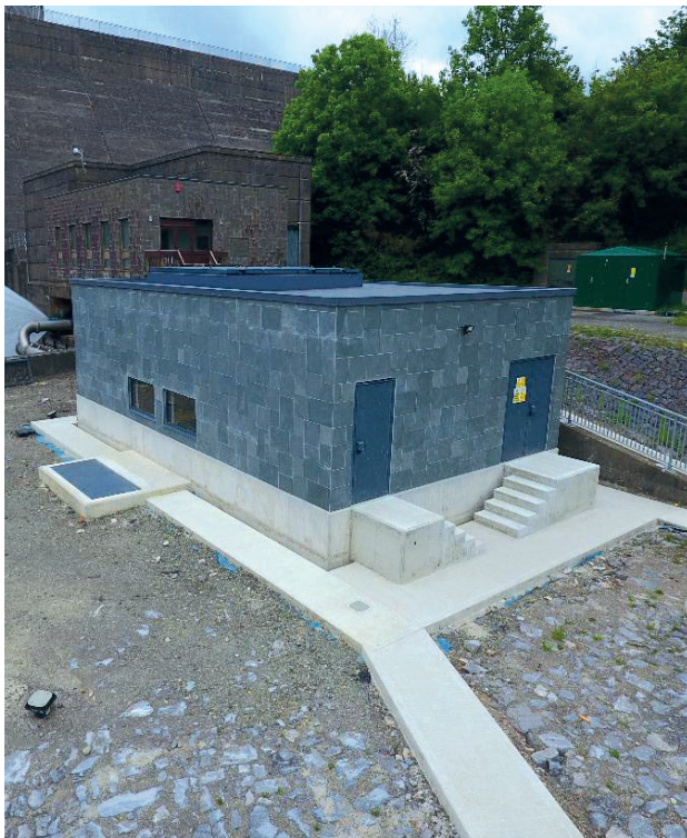
The Llys Y Fran project near Haverfordwest – a hydro scheme that controls the flow release to the Afon Syfynwy in order to support abstraction at Dyr Cymru's Canaston Bridge pumping station. The project has an installed capacity of up to 250 kW and the power generated will be exported to the grid via an existing connection.
