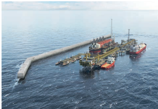
The Greater Tortue Ahmeyim project will produce gas from an ultra-deepwater subsea system and mid-water floating production, storage and offloading vessel (left), which will process the gas for transfer to a floating liquefied natural gas facility at a nearshore hub located on the Senegal/Mauritania maritime border.
