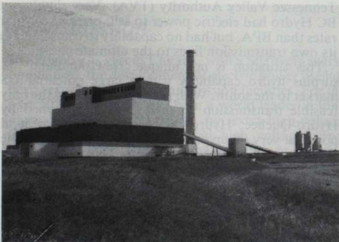
The coal-fired Sheerness station is the first joint venture between Alberta's two investor-owned utilities — Alberta Power, which is the managing owner, and TransAlta Utilities Corporation. The station is located near Drumheller and uses surface-mined coal from an adjoining field. The first of two 380MW units is in service and cost Cdn$630 M. The stack is 132 m high. (Photo courtesy of Alberta Power)
