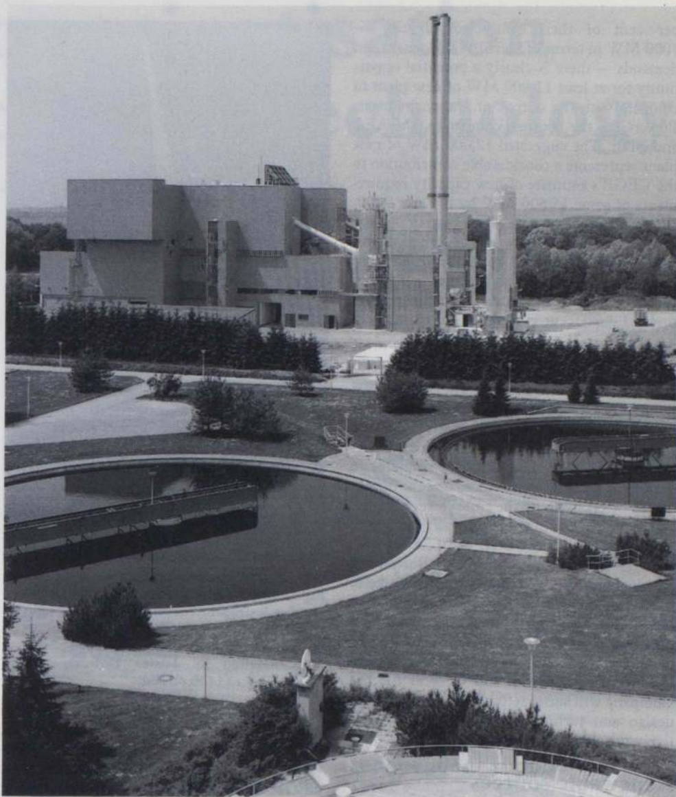
Fig. 3: a modern refuse incineration CHP plant located near Munich, West Germany.
