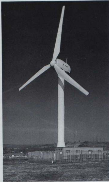
Fig. 2: the three-bladed 300 kW wind turbine generator currently operating on a CEGB site at Carmarthen Bay, South Wales. The machine was designed, built and installed by James Howden and Company Ltd of Scotland.
