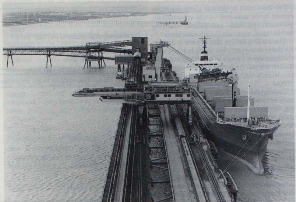
The modern, automatic coal conveying and loading systems are reflected in this picture of loading operations at British Coal's Immingham Bulk Terminal at South Killingholme, Humberside.
