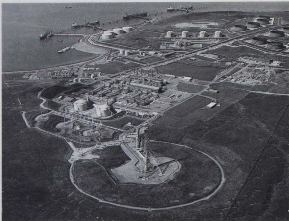
The process plant at Sullom Voe Terminal, Shetland.
