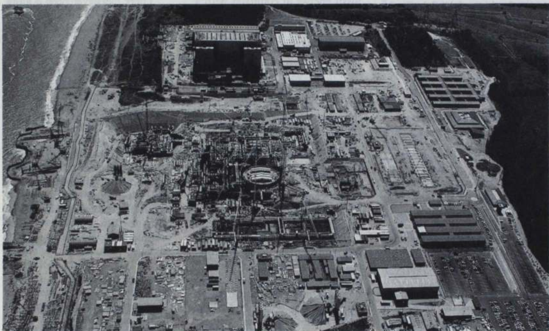
A recent aerial photograph showing the Sizewell B construction site in the foreground and the Sizewell A magnox nuclear power station in the background.
