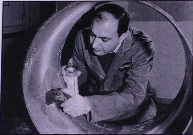
A candidate carries out a magnetic particle inspection of a weld root on a section of pipeline.
