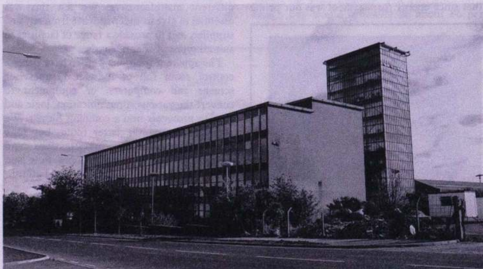
Emstar's energy management system has contributed to over 65 per cent energy savings for NEI IRD, achieving a carefully controlled balance between the heating and cooling systems in the building.
