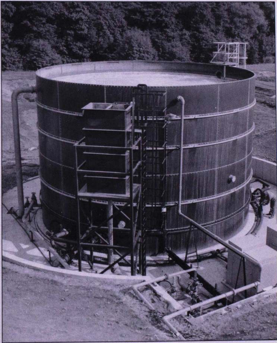
Venturi aeration systems reduce biological oxygen demand.
