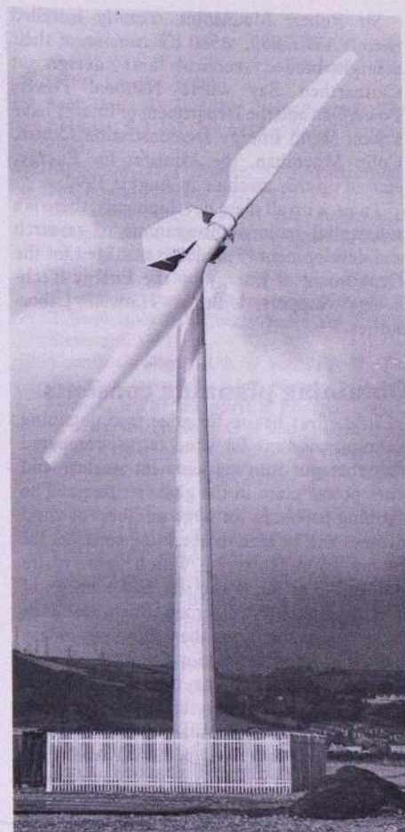
The two-bladed, 300kW demonstration wind turbine generator designed by Wind Energy Group Ltd and located at Carmarthen Bay, S. Wales.
