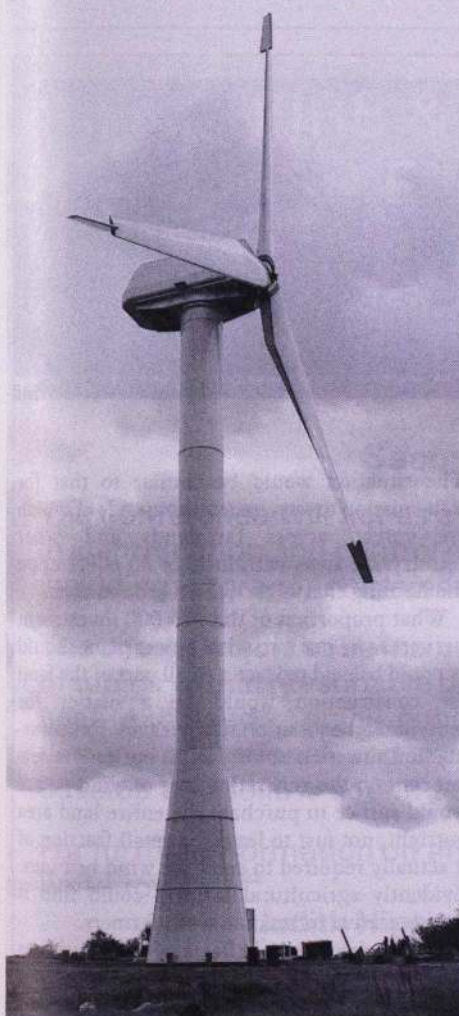
The recently-inaugurated Howden 1MW wind turbine generator at Richborough in Kent.
