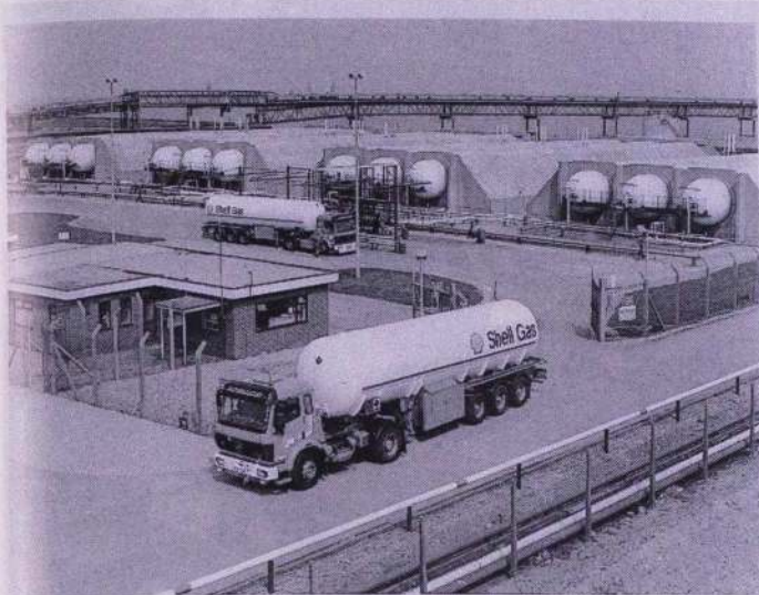
ShellGas import facility at Immingham.
